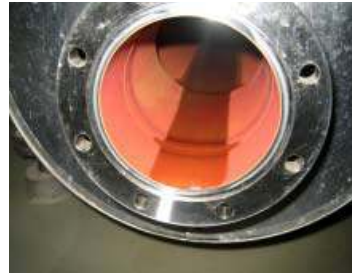
Left: Red-brown Rouge layer in WFI-tube system (material 316L)
