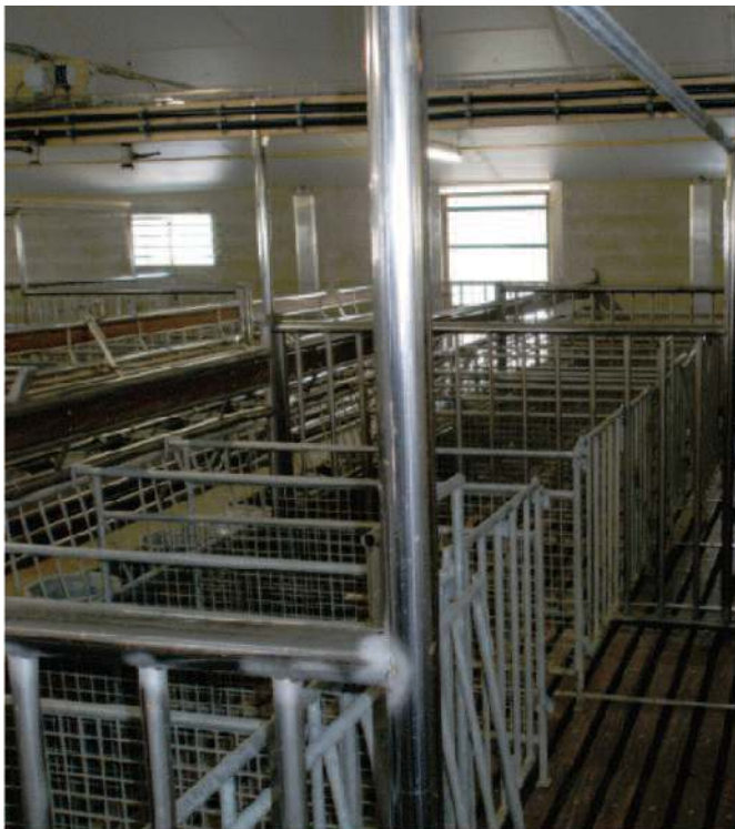
Fig. 8. The annealing colours on the welded joints have been removed with dry ice which includes an abrasive additive. This results in milky-white patches that are, however, resistant to corrosion.
